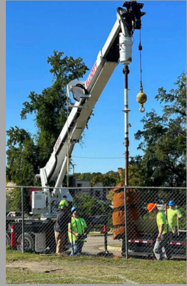
Field lights being installed in outdoor field.
